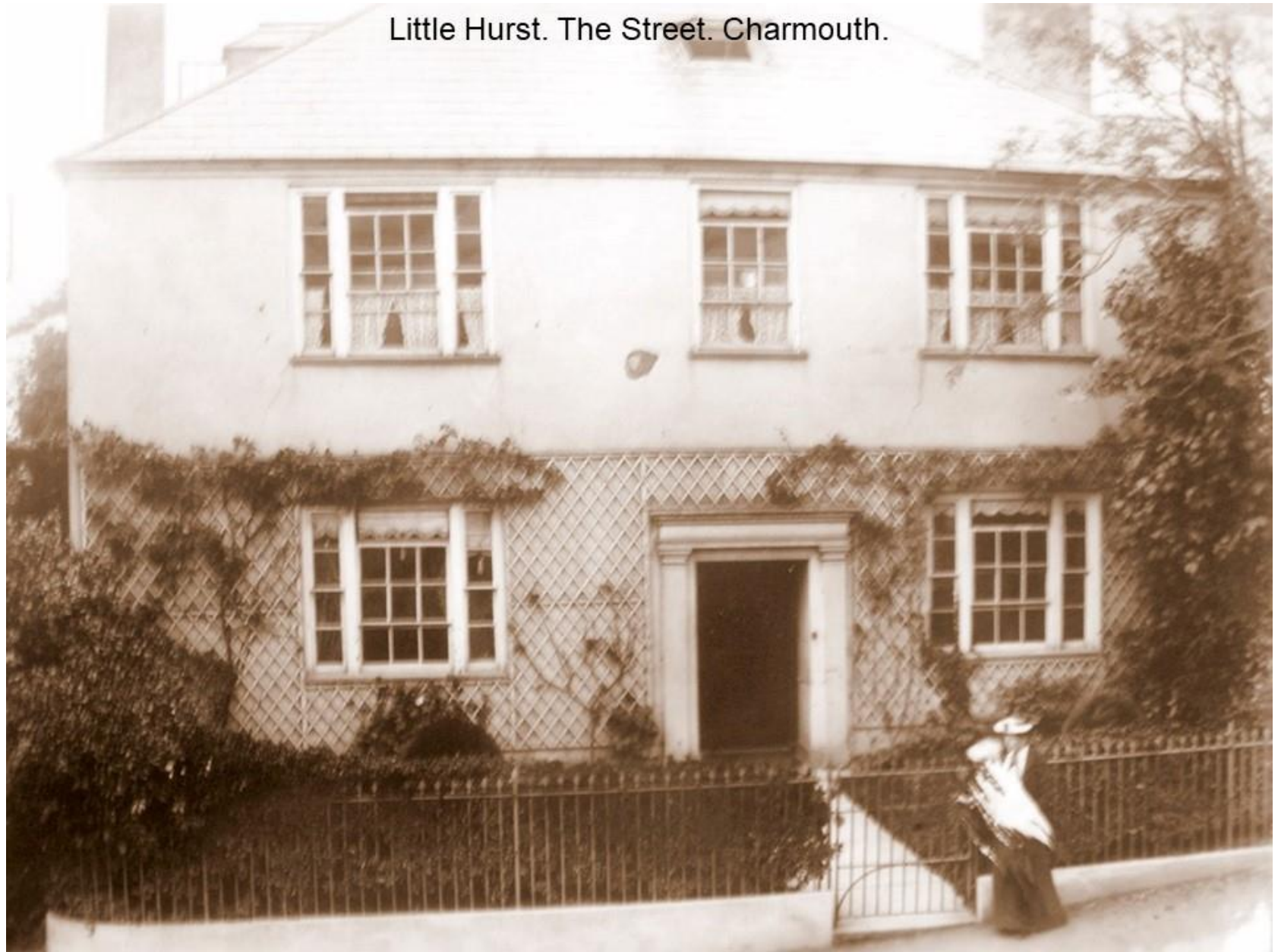
Robert Culverwell would have owned this house in 1803. He was very wealthy and it was one of a number that he rented. It was probably leased by Joseph Hackman who was described as a Gentleman and was buried in the Church in 1817 aged 90.
